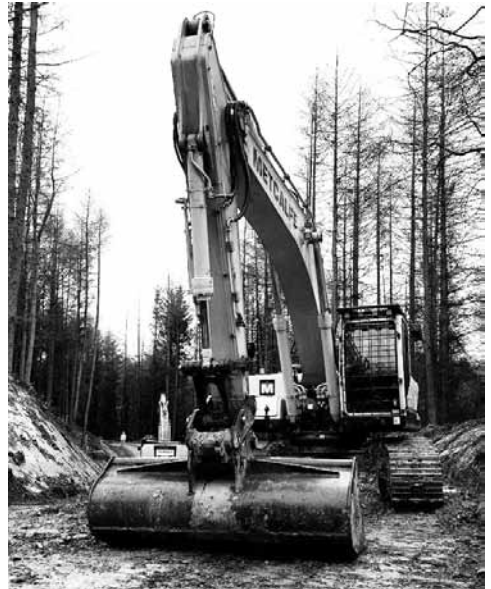
Site access road under construction.
